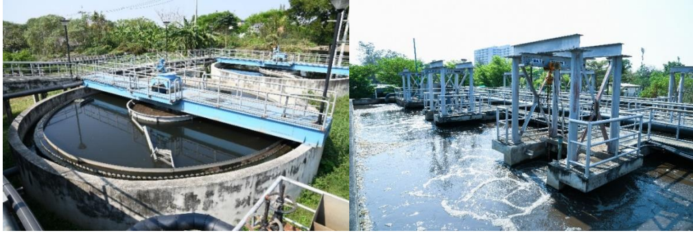
Wastewater treatment system of Salaya campus
