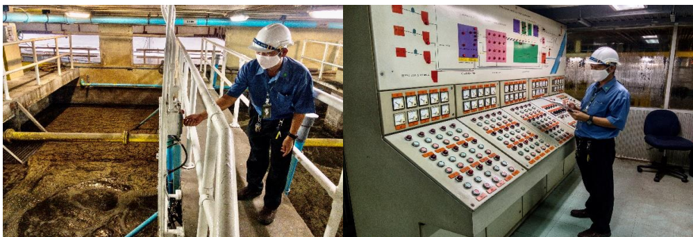
Wastewater system of the Faculty of Medicine Siriraj Hospital
